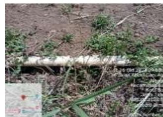
Gambar : 10 Pipa Lateral
